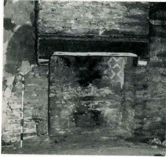
Plate 3b. Second floor west fireplace showing 'sgraffito' plaster decoration.
